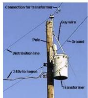
• Operates on the principle that a current in one coil (primary) induces a current in another coil (secondary).
